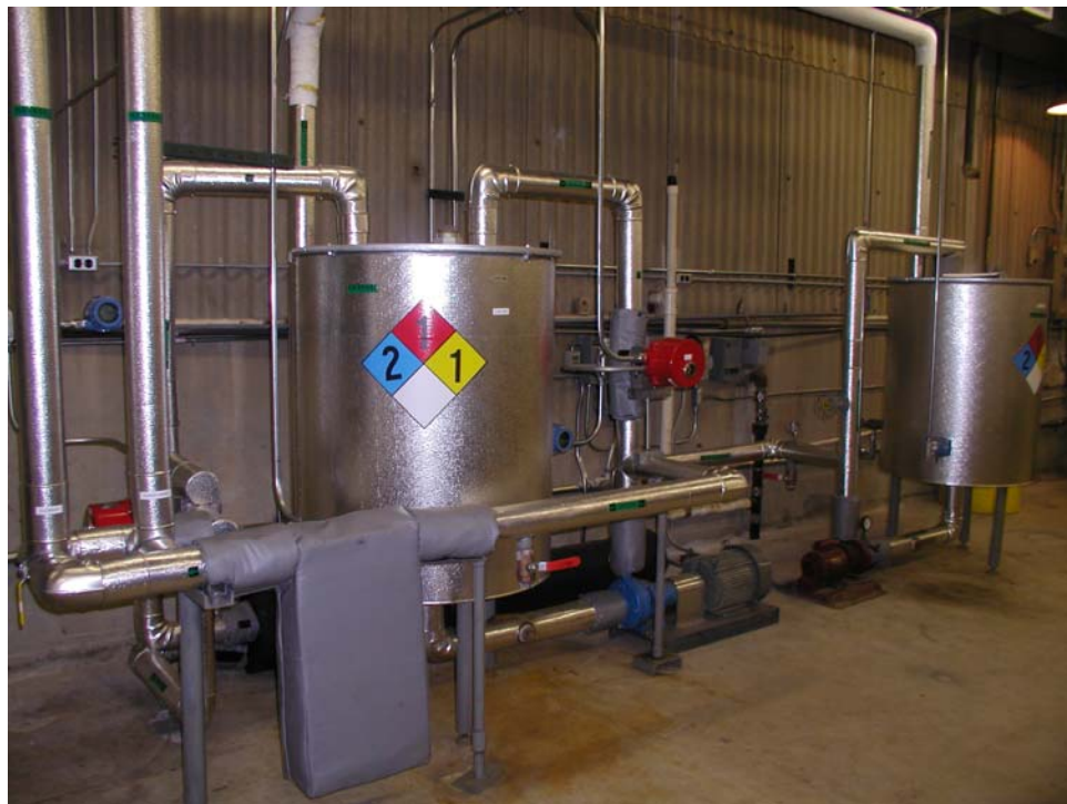
Figure 5 – Photograph of Glycol System
